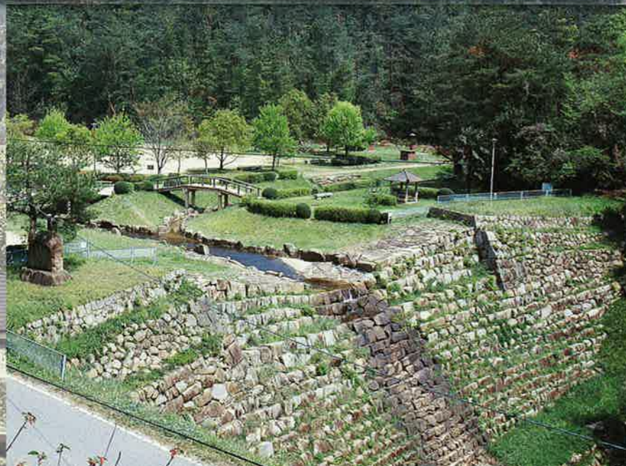
Dodo Park and Check Dam No. 6
