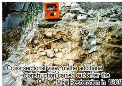
Condition of the Dam Face after Excavation
