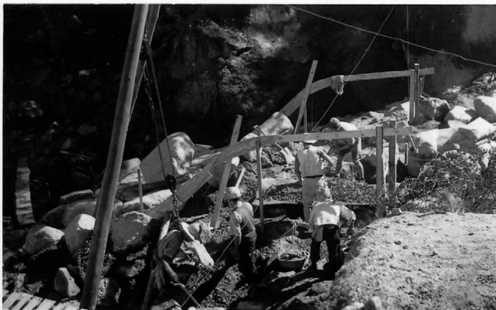
Construction status of the No.5 dam in 1949 (※1)
