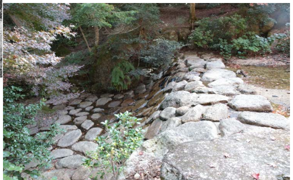
Current No.5 dam
