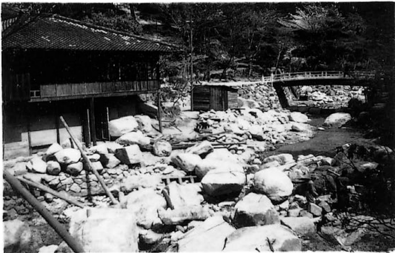
Damage downstream from Momiji Bridge (※1)
