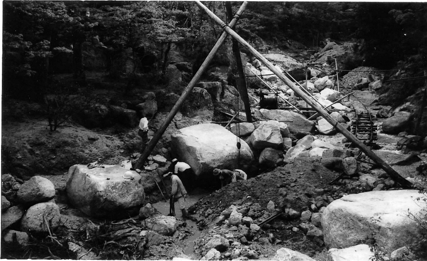
Construction status of the channel works upstream from Momiji Bridge (※1)
